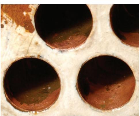
**Figure 11** - After the cleaning, the chiller's heat exchange efficiency was completely restored
